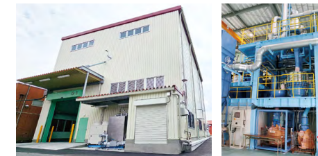
New fire-extinguishing agent recycling plant
